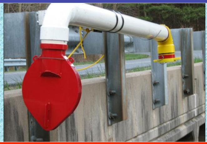
A Kochek teardrop strainer is used in most all of our swiveling standpipe systems. The strainer's low profile design allows it to be used in shallow, moving water.
