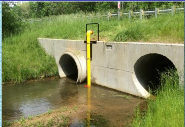
This installation used a modified, saddle mount bracket to secure the standpipe. No holes were drilled into the concrete wall.
