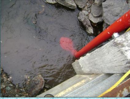
The folks in Austerlitz, NY were able to flow 1000+ gpm from this installation using a two-person deployment team.
