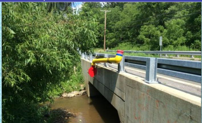
This dry hydrant uses a swiveling standpipe type of design on a traditional guard rail type of bridge wall. The pipe is stowed on a bit of an angle in order to ensure drainage during the winter.
